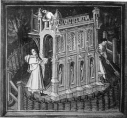
BUILDING THE CHAPEL ST. FREMUND
